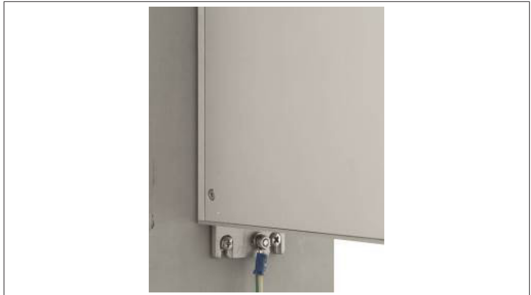
Figure 28: Grounding detail
