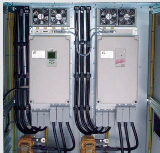
560 kW P-housing cascaded
